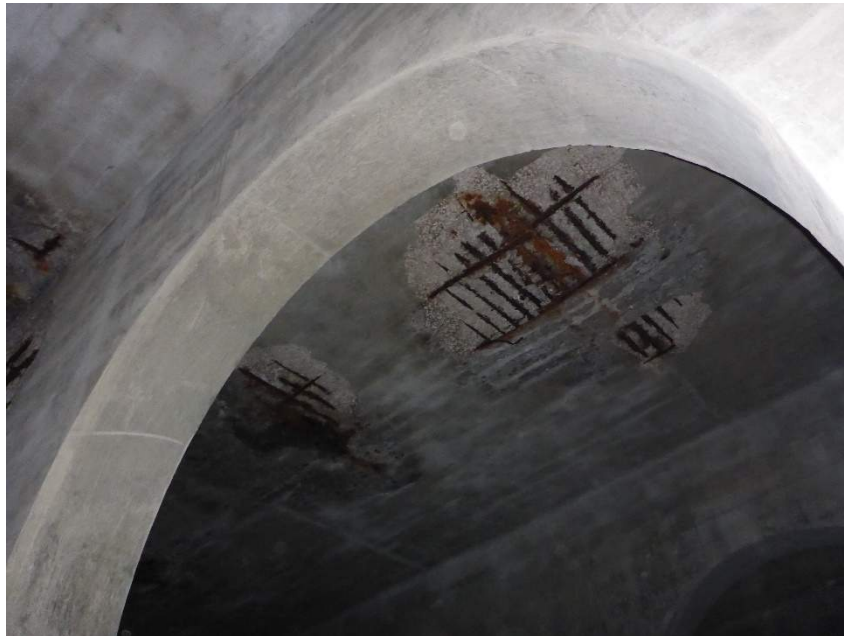
Photo 4: Typical Spalls with Deteriorated Rebar on the Deck in the East Approach Spans (2024 Inspection Photo)
