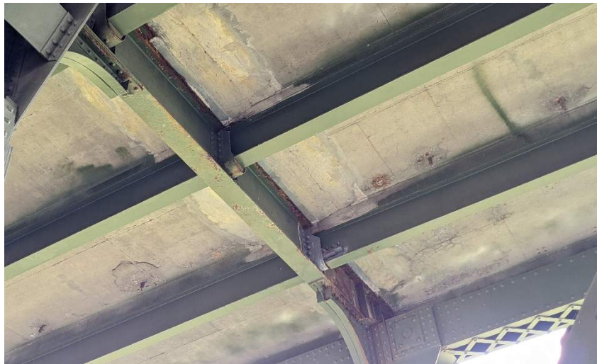
Photo 10: Stringer-Floorbeam Connection Repair
