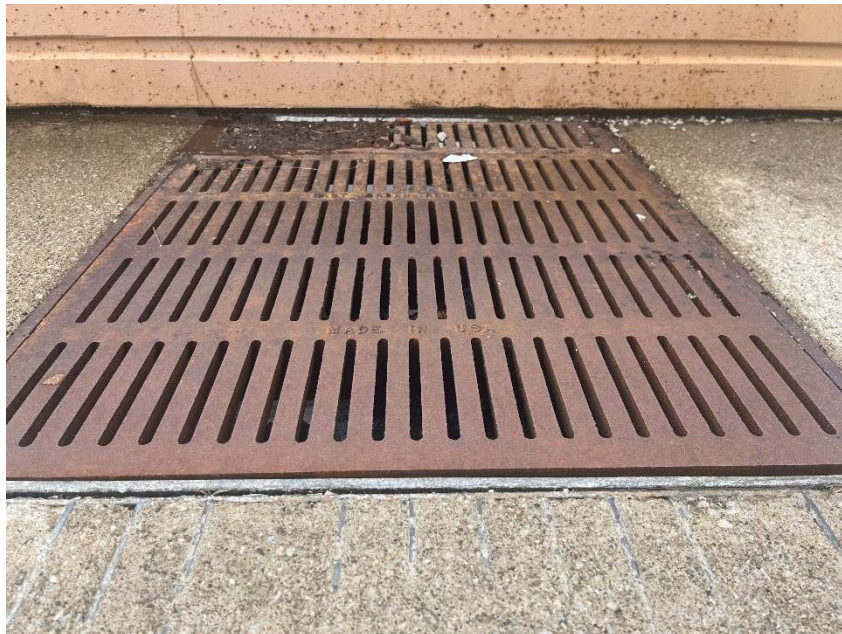
Photo 5: Typical Clogged Drainage Recesses Covered by Grates in the North Sidewalk
