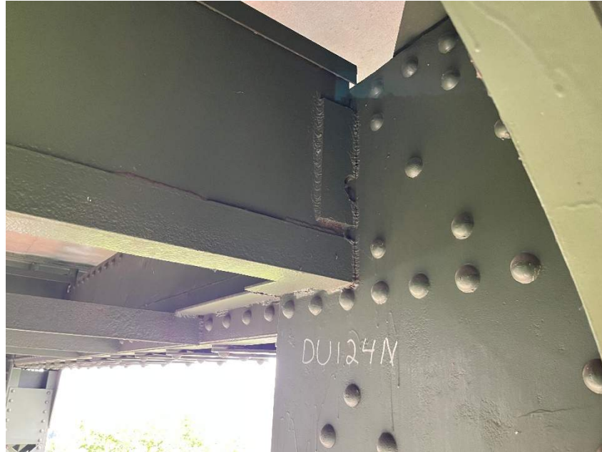
Photo 12: Cracked Weld of the Abandoned Utility Attachment at U4-U5 of the Span 6-7-8 South Exterior Truss
