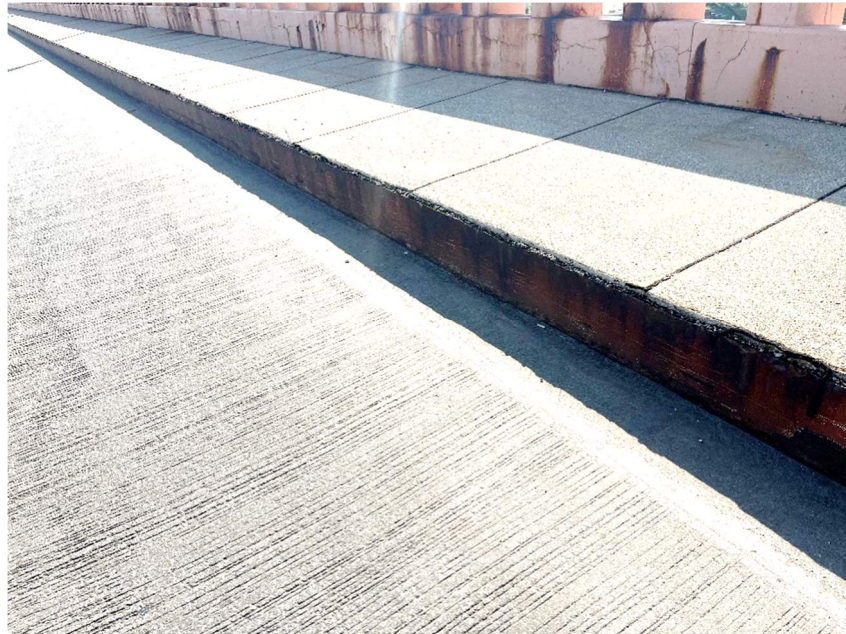
Photo 6: Typical Rusting Steel Curb Plate on South Sidewalk
