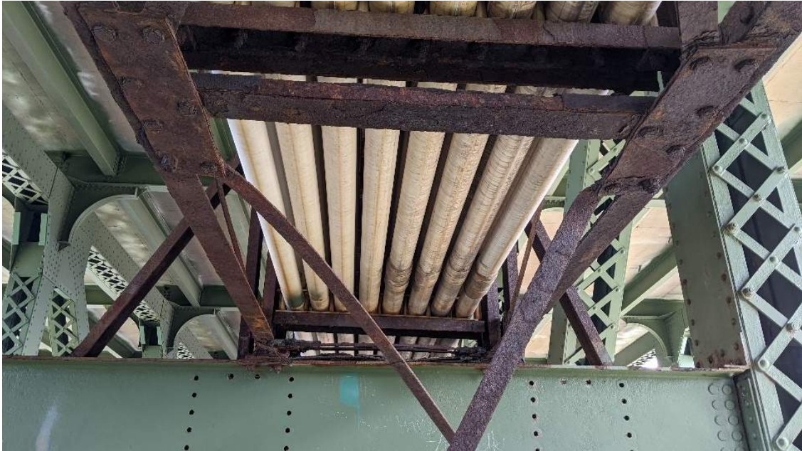
Photo 34: Typical Deteriorated PVC Conduit Truss with Broken and Warped Gusset Plates
