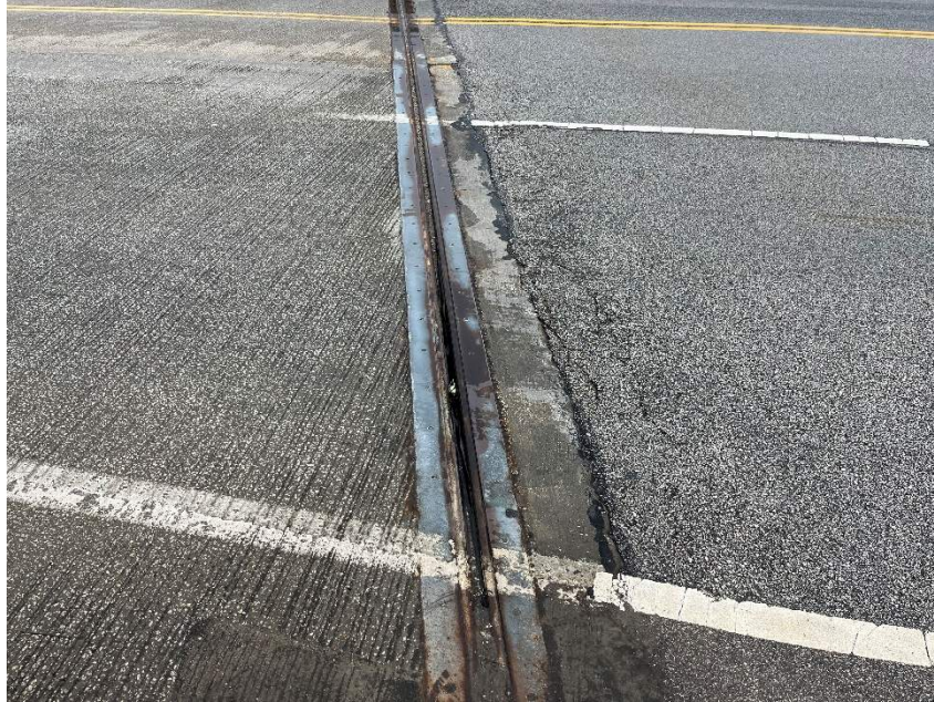
Photo 25: Missing Length of Joint Material in Expansion Joint 17
