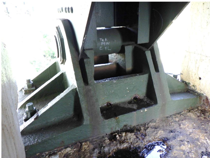
Photo 21: Standing Water Around Bearing at L14 North Exterior Truss
