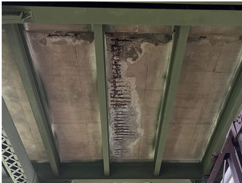
Photo 2: Large Spall with Deteriorated Rebar on the Deck in Span 12
