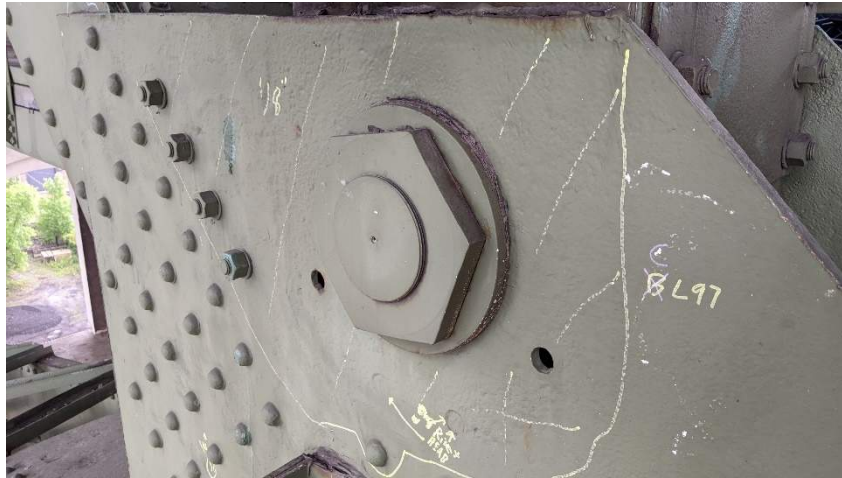
Photo 14: Gusset Plate at L0 in Span 4 of South Interior Truss
