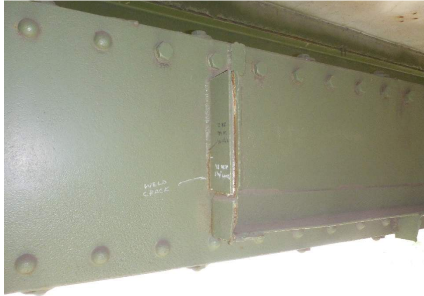
Photo 15: Weld Crack at U0-U1 in Span 10 of South Exterior Truss (2024 Inspection Photo)
