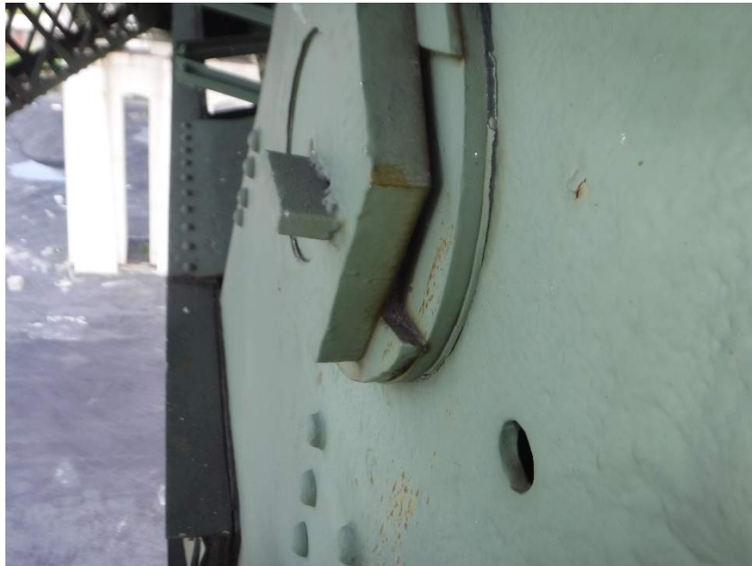
Photo 13: Recessed Pin at L17 in Span 9 of North Interior Truss
