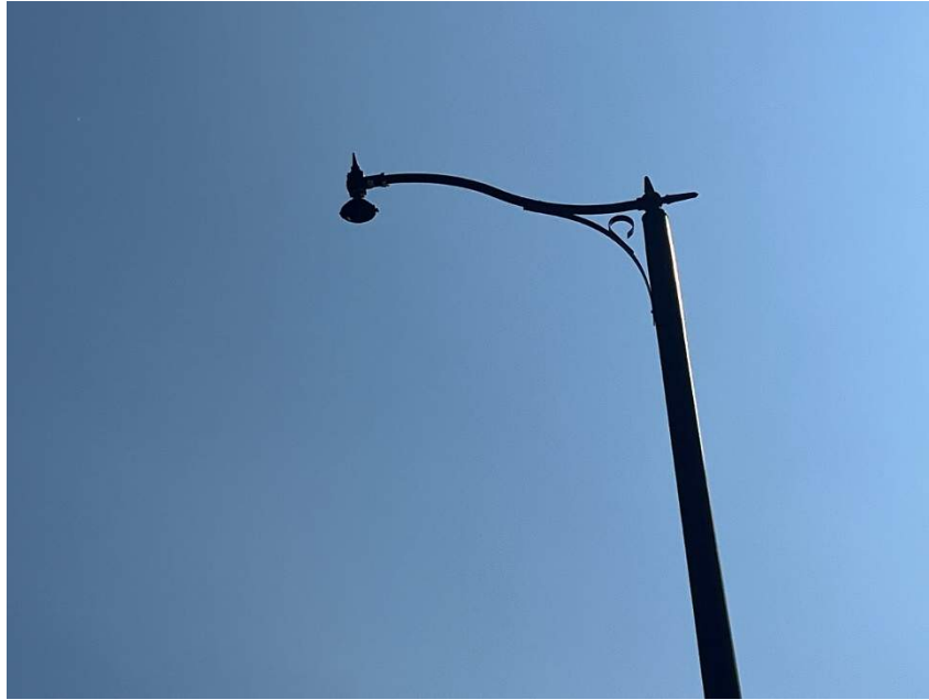
Photo 39: Street Light Missing Globe Outside of South Railing in Span 7
