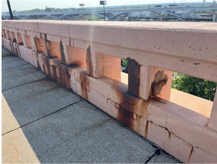
Photo 23: Typical Deteriorated Exterior Railing
