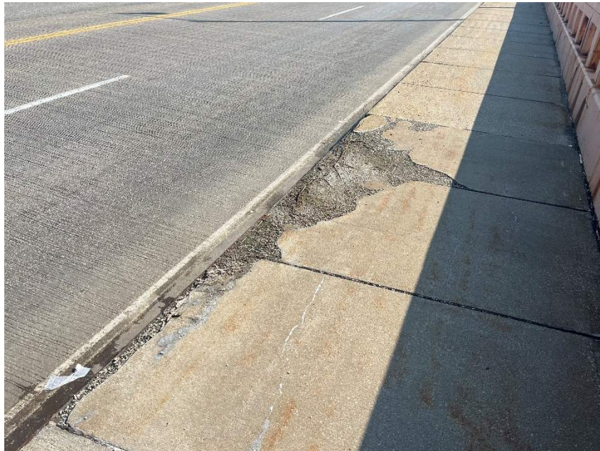
Photo 8: Spall with Deteriorated Reinforcing in Span 7 of South Sidewalk
