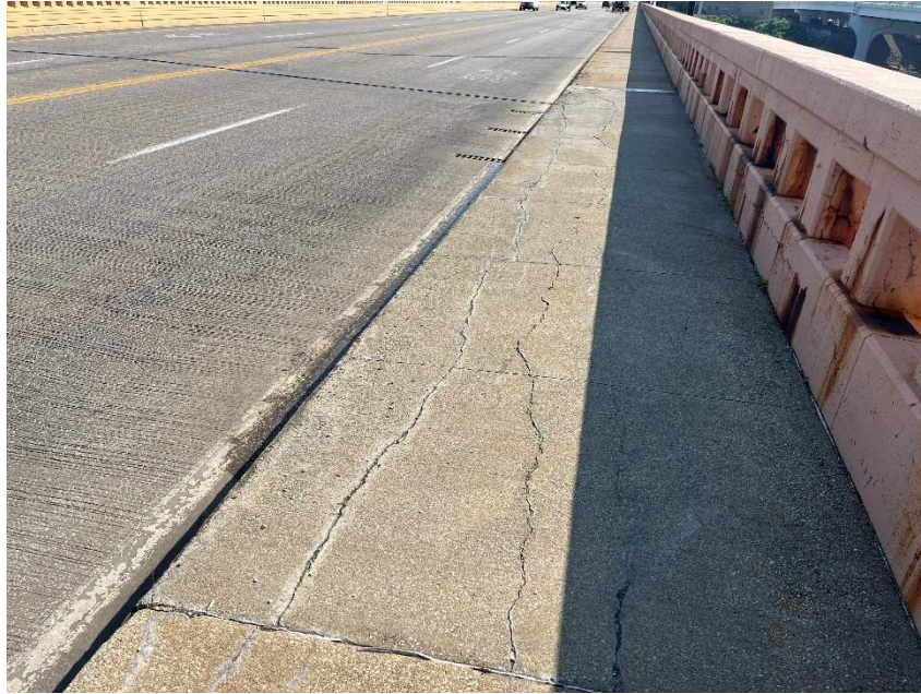
Photo 7: Typical Cracks on Sidewalks
