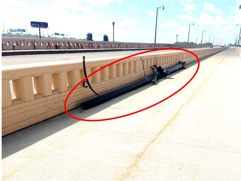
Photo 37: Removed Street Light Pole Laying Against North Interior Railing in Span 3
