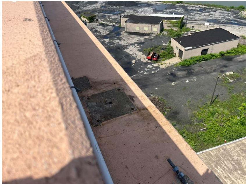
Photo 38: Missing Street Light Pole Outside of North Railing in Span 6
