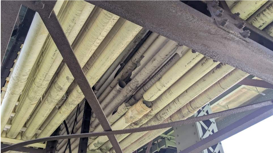
Photo 33: Typical Damaged PVC Conduits
