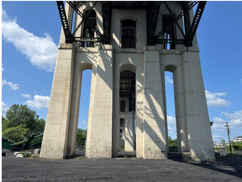
Photo 17: Scraping Damage of East Faces of Columns of Pier 7
