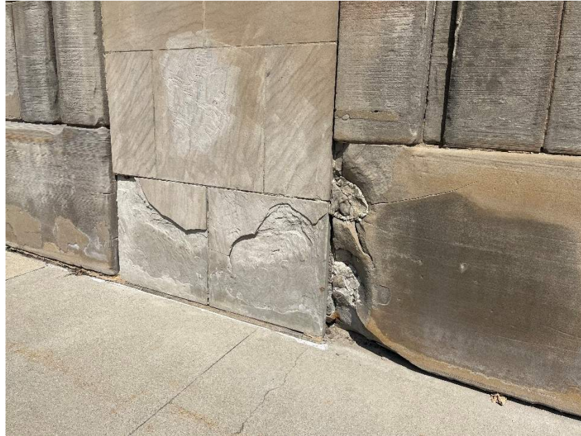
Photo 22: Typical Spalls on Northeast Decorative Pylon
