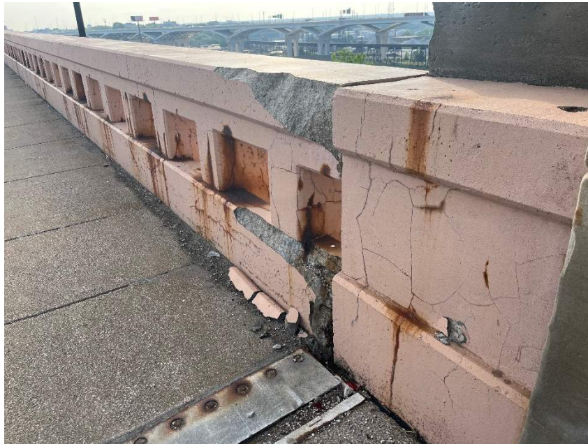
Photo 31: Typical Cracks, Spalls, and Rusting Staining on Approach Railing
