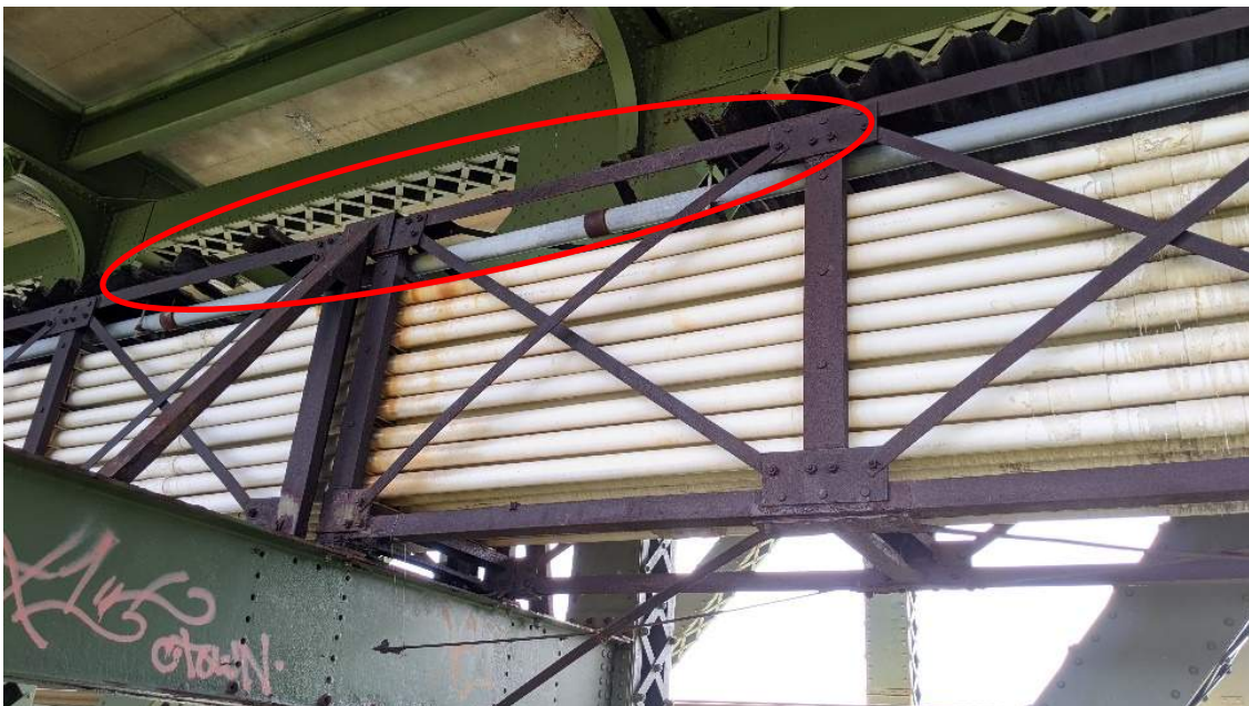
Photo 35: Typical Deteriorated Corrugated Roof For PVC Conduits Under Deck Joints
