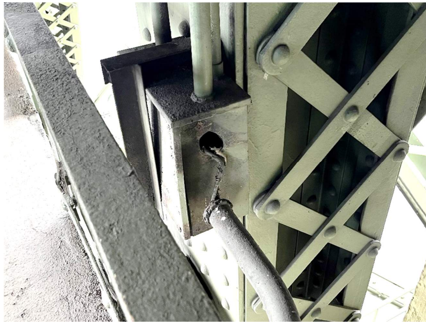
Photo 32: Electrical Conduit Detached From Utility Box in Span 7
