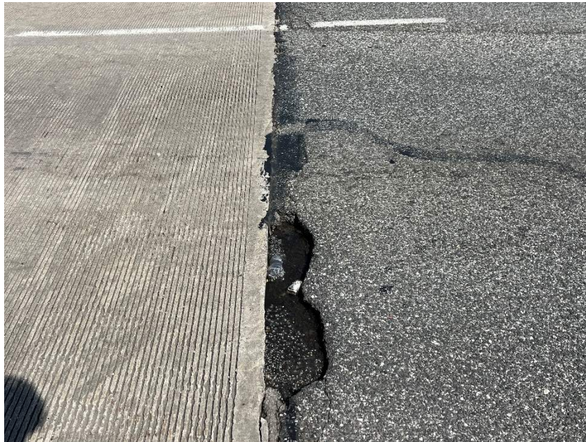
Photo 30: Large Pothole at Joint Between East Approach Slab and Approach Pavement
