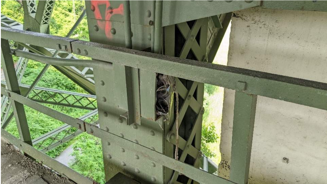
Photo 36: Deformed Junction Box For Electrical Conduit with Deformed Cover Plate in Span 13
