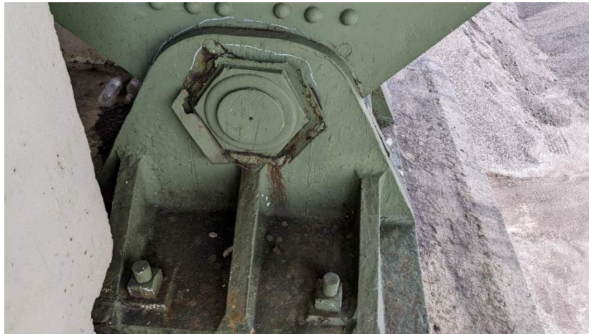
Photo 24: Typical Section Loss on Pin and Surface Corrosion on Bearing
