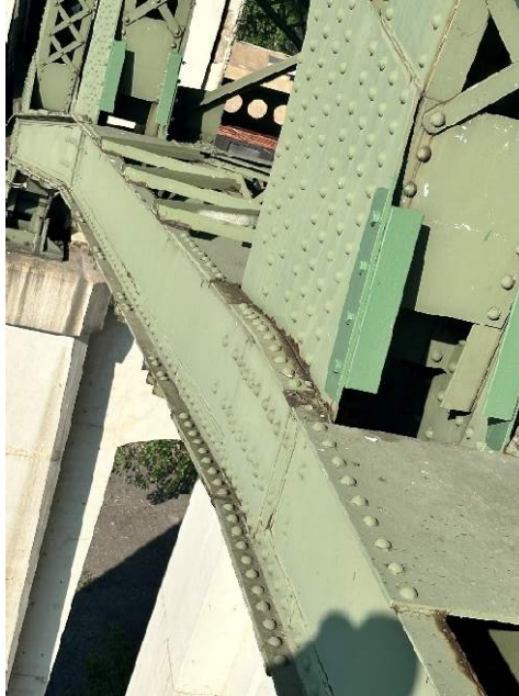
Photo 16: Typical Fading and Loss of Pigment of Paint
