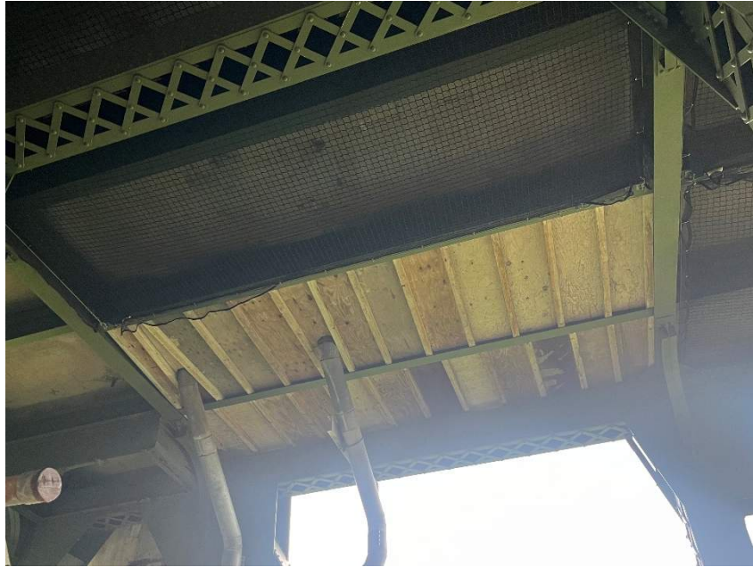
Photo 3: Typical Netting and Falsework Below the Deck
