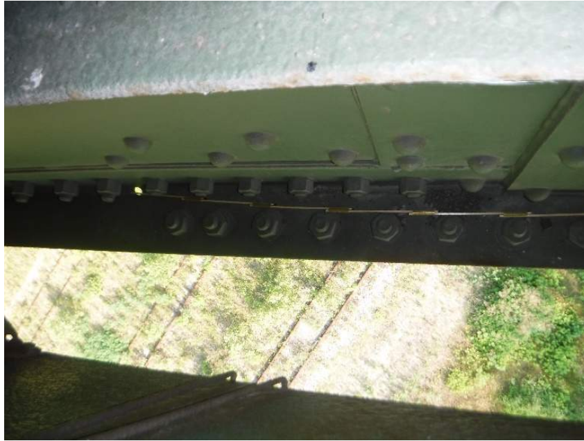
Photo 11: Crack Arrest Hole at Bottom Flange L3-L4 5" West of the West end of the Crack in the South Lower Flange angle at L4 of North Interior Truss
