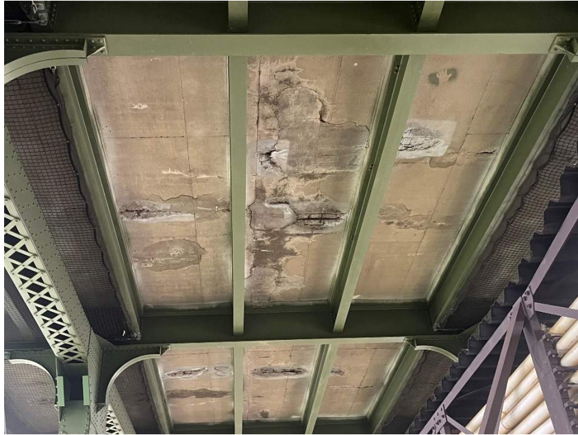
Photo 1: Typical Spalls with Exposed Rebar, Delaminations, Cracks with Efflorescence, and Failing Patches on the Deck
