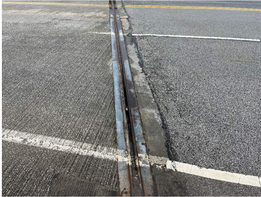
Photo 26: Damaged Seal and Debris in Expansion Joint 18
