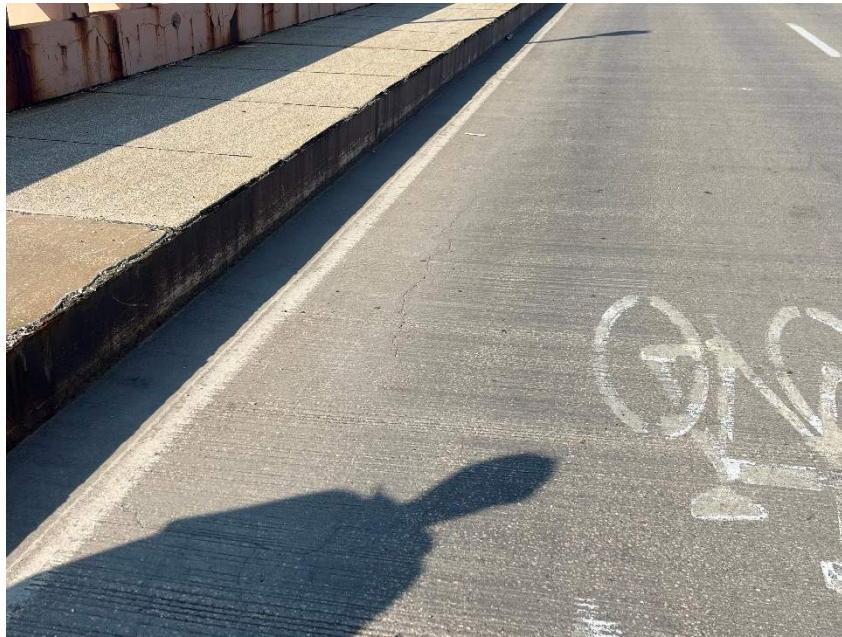
Photo 9: Typical Minor Cracks in Wearing Surface
